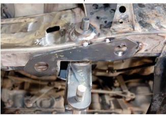
**STEP 28** Finish welding the bottom support plate.
